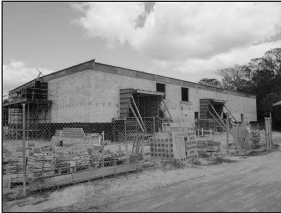
New Water Treatment Plant Being Built
